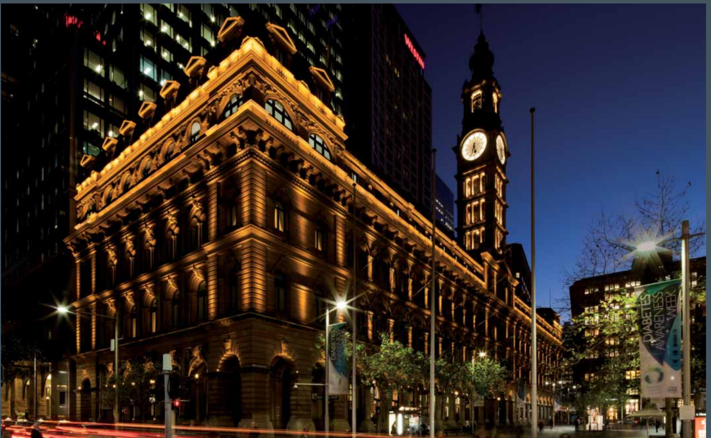
No 1 Martin Place, Sydney/Australia Lighting design: Point of View, Melbourne/Sydney
