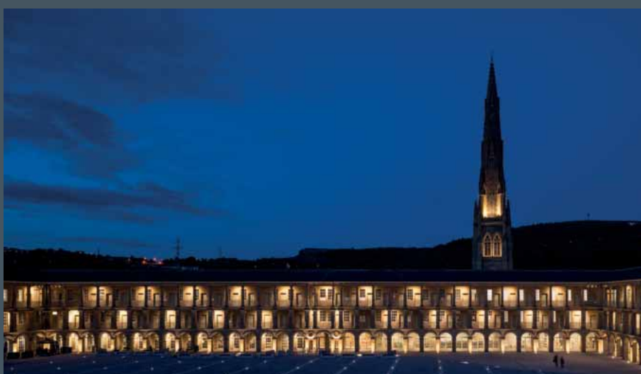
Piece Hall, Halifax/UK Lighting design: Buro Happold Lighting, Edinburgh
