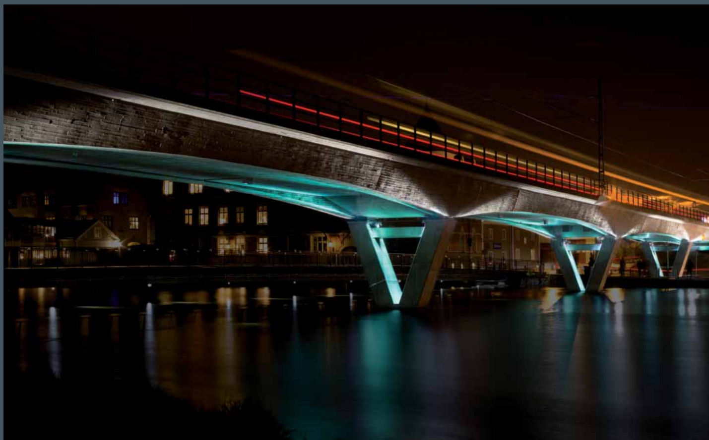
Railway Bridge, Eskilstuna/Sweden Lighting design: ÅF Lighting, Stockholm Photo by Sten Jansin
